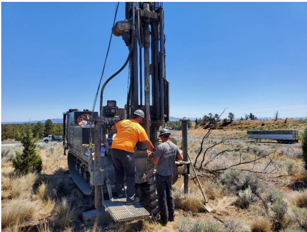
Geotechnical explorations performed with track-mounted CME-75 by Western States Soil Conservation Inc.
