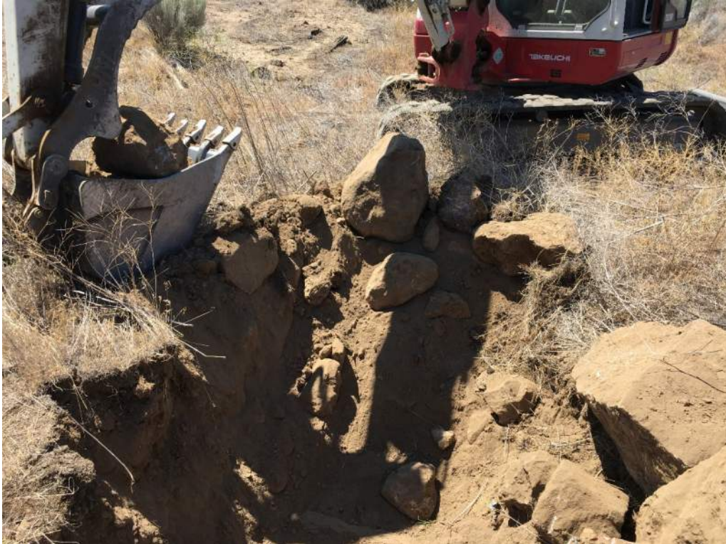
TP-02 spoils with boulders and refuse.
