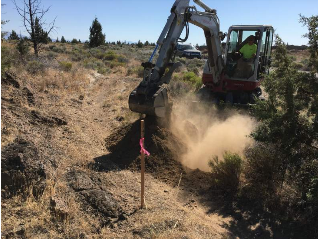
Test pit operation using mini-excavator operated by Terry Shine Excavation.
