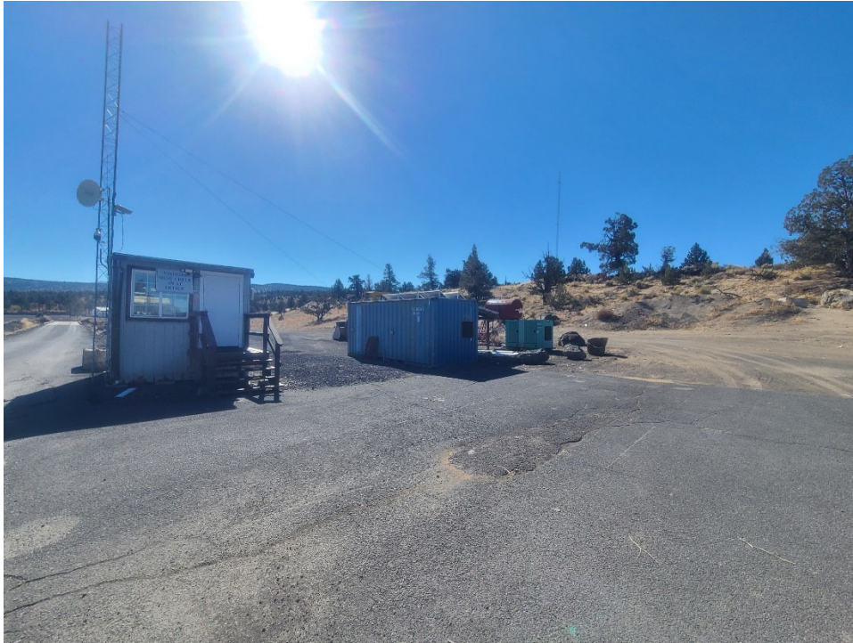
Photograph 7. Infrastructure at entrance.
