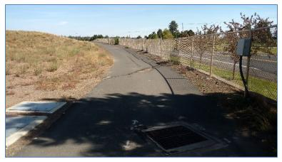
SA has reviewed the present condition of the perimeter road subgrade adjacent Rickard Road where it is apparent that the road is constructed on a subgrade composed of MSW. The asphalt surface is distressed as a result of consolidation and displays swales and wide cracks indicative of an unstable subgrade. Further, the distress has disrupted the design drainage pattern.
