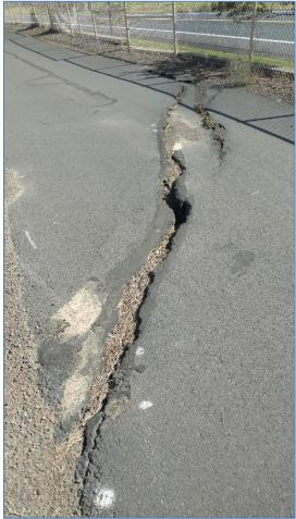
reinforcment grid is believed to be located just below the pavement subgrade. Hence, care must be observed to prevent damage to the horizontal reinforcement during the reconstruction.
