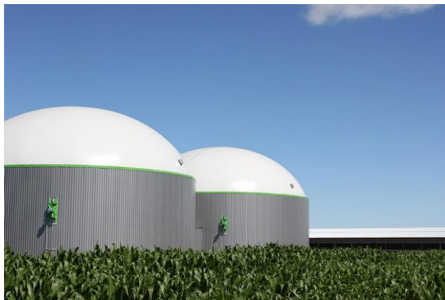
Figure 6-14: Typical CSTR AD System
