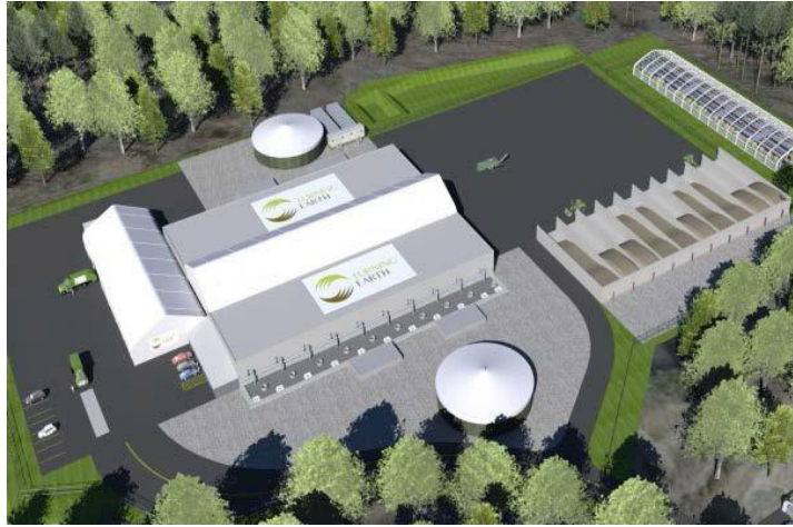
Figure 6-18: High Solids AD with Integral Composting Operation (Image courtesy of Turning Earth, LLC)
