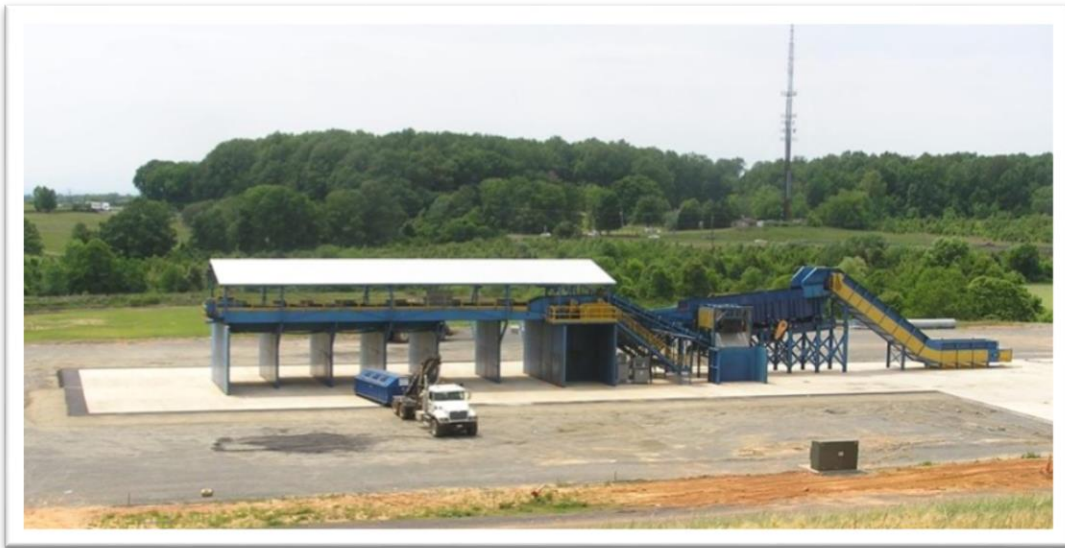
Figure 4-7: Example C/D Processing Infrastructure
