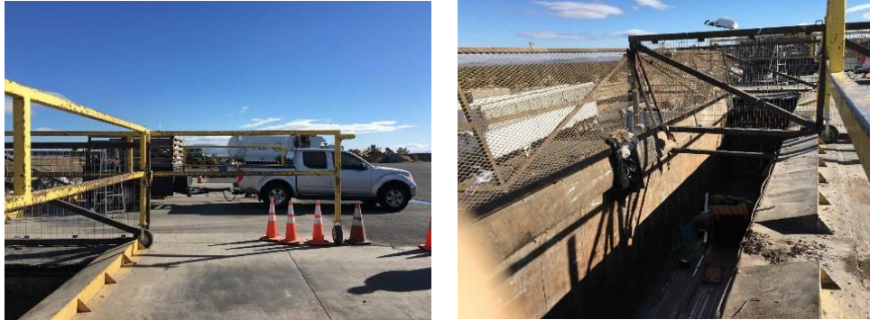
Figure 5-6: Negus Transfer Station Safety Features
