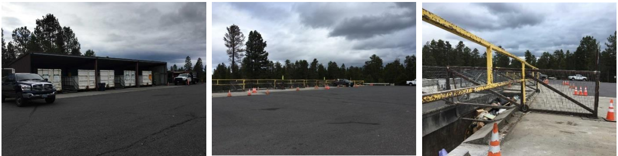
Figure 5-7: Southwest Transfer Station
