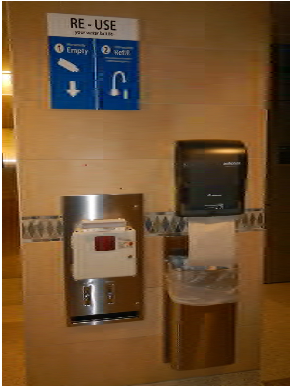
Figure 36 : Restroom signage encouraging passengers to reuse water bottles
