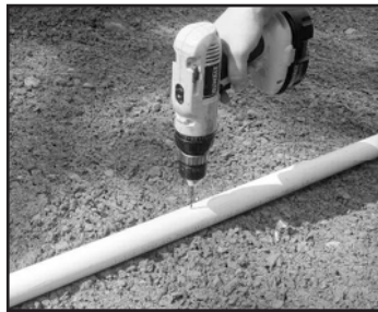
1. Drill hole in pipe.
