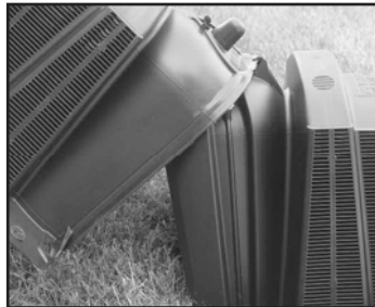
8. Attach endcap to chamber.
