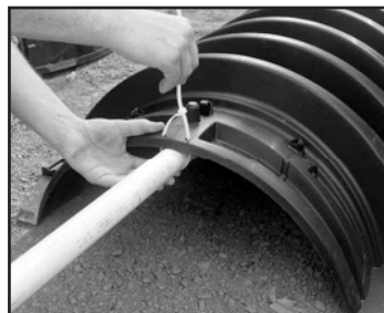
5. Secure pipe to chamber.
