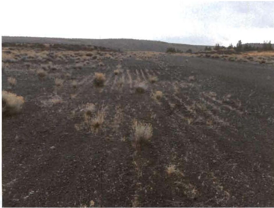
View looking south along aggregate-covered access road. Note sparse range grass growth in furrows from reclamation seeding.
